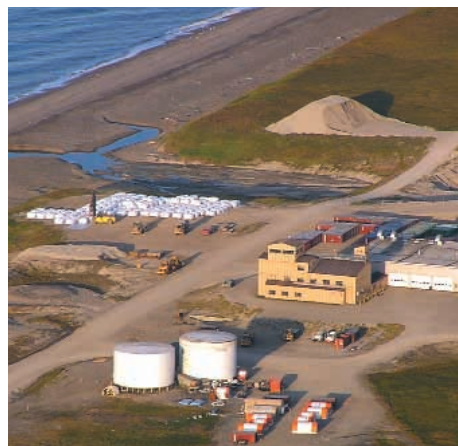
Project site near Cape Lisburne, Alaska, where our Lift Liners™ were used to package and transport contaminated soil.
